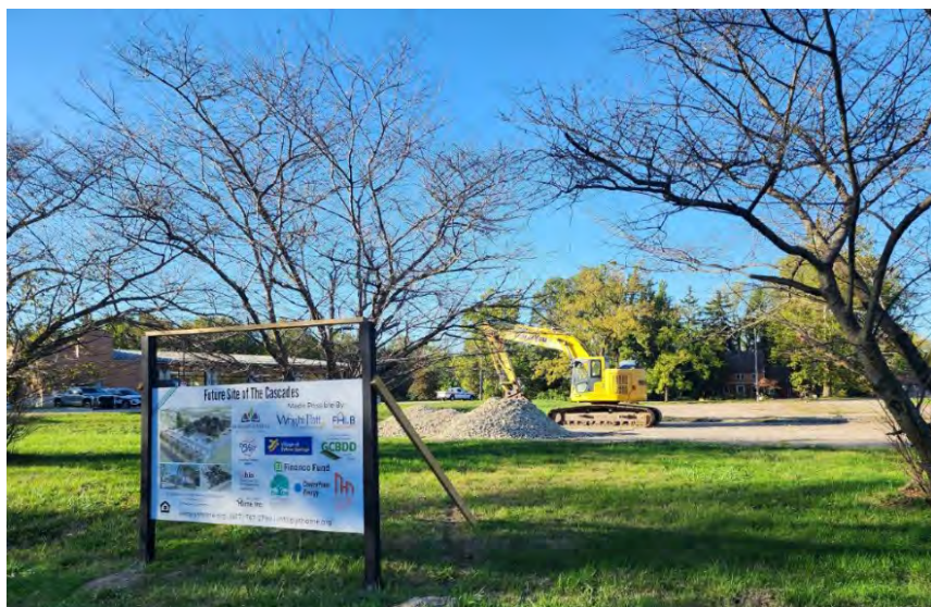
Construction begins at The Cascades – October 2024
